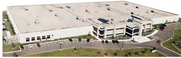
Headquartered in Anoka, Minnesota, in a 300,000 sq. ft. state-of-the-art facility.
